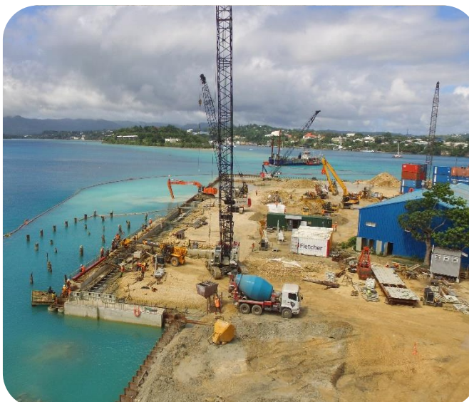
Pouring Concrete for Coping Beam at Wharf
