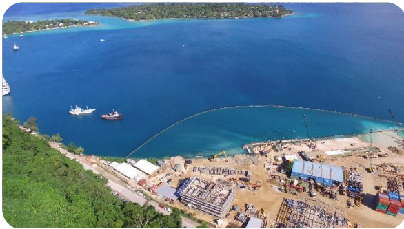
Silt Fence Installation
