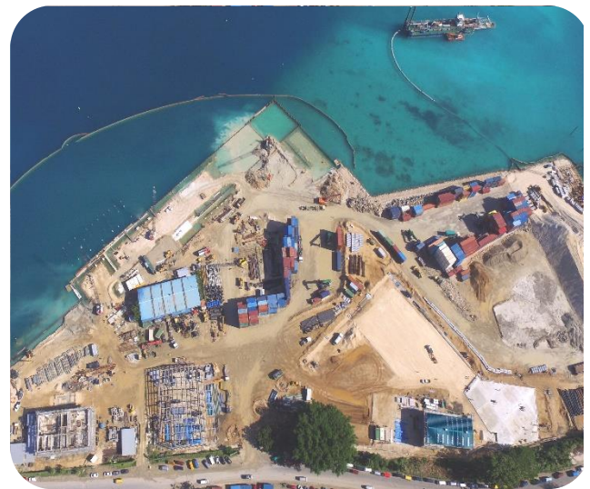
Present Site Situation
